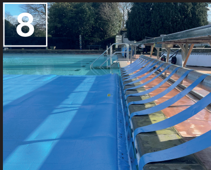
Step 9. Attaching the straps to the reel system and wind wires to the pool side. The 4mm wire is attached to the pool wall using tough stainless-steel fixings.
